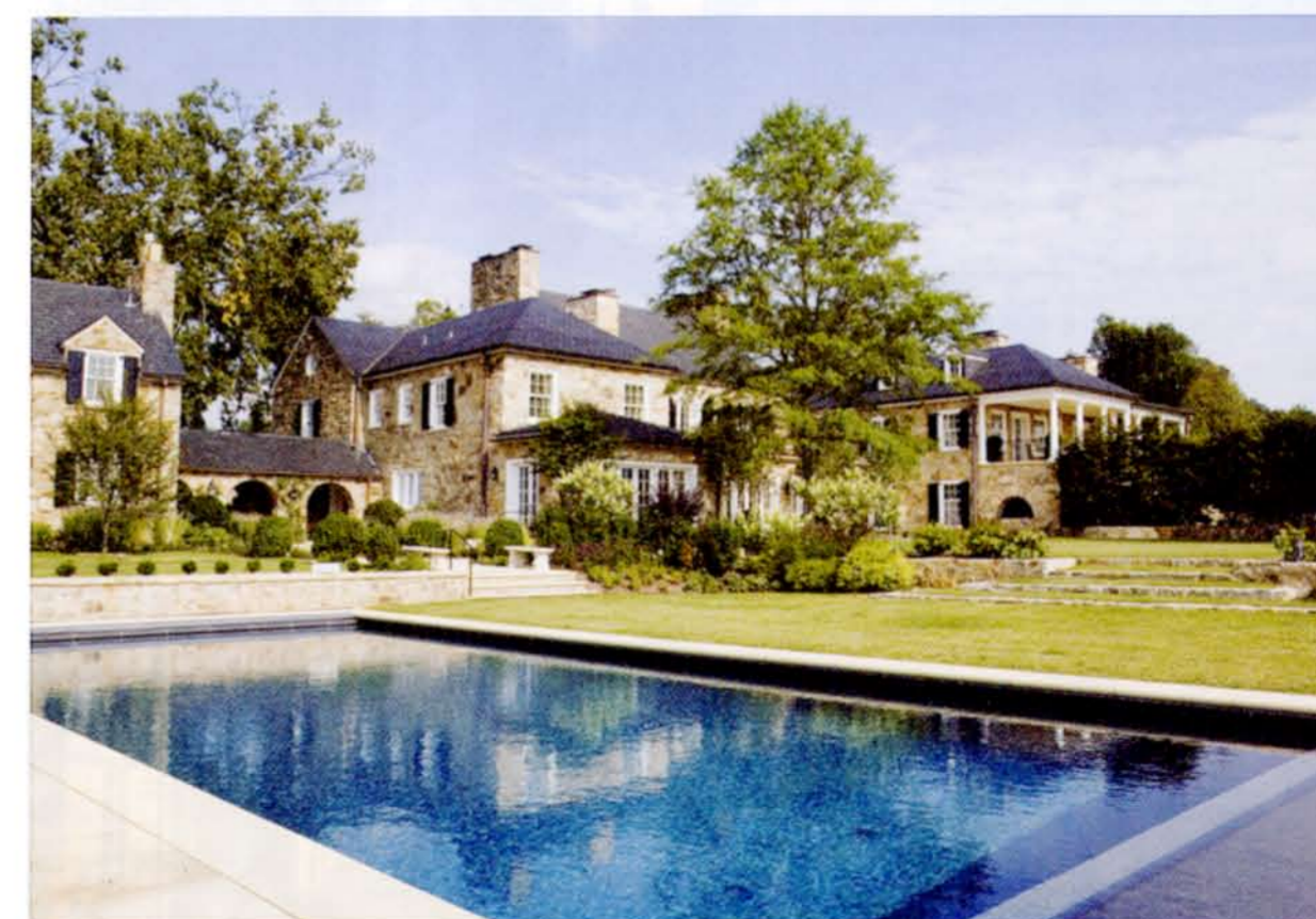
This overall view of the rear of the house from the pool reveals the expansiveness of the home, with the children’s bedroom and loggia at the left, the formal center portion of the home and then the master suite with the colonnaded terrace.
